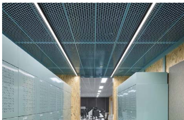
Undertak i perforerad metall som tillåter bakomliggande akustikabsorbenter. People's Choice Credit Union headquarters office. Woods Bagot. Foto David Sievers
